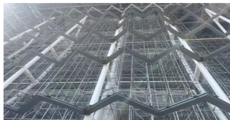
Figure 4 Installation of Broken Line Beams
