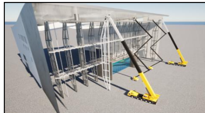
Figure 3 Installation of Fish-Belly Steel Trusses
