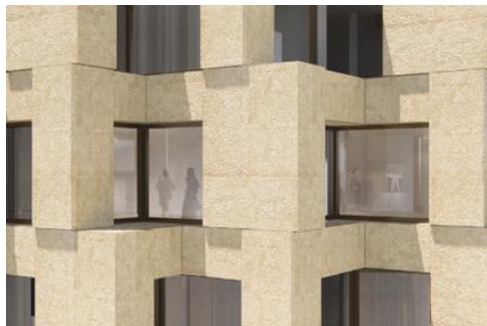
Figure 1 Imitation stone concrete hanging board curtain wall
