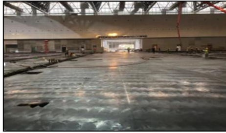
Figure 2: Finishing the Surface
