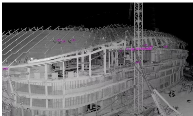
Figure 7 Curtain wall three-dimensional scanning site
