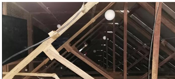
Figure 13 Three-dimensional scanning station distribution map of ballast steel structure
