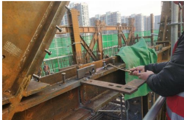
Figure 2 Welding Preheating Treatment
