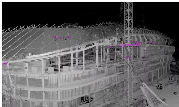
**Figure 7** Curtain wall three-dimensional scanning site
