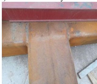
Figure 8 Steel Platform Welding
