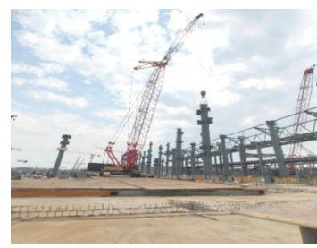
Figure 9 Roadbed Box Full Paving
