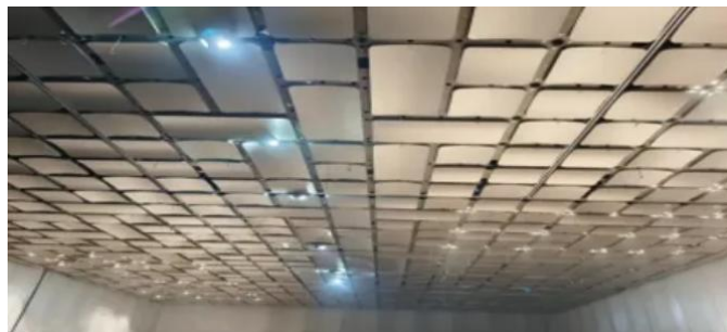
Figure 9 Rendering of Unitized Installation of Curved Honeycomb Aluminum Ceiling
