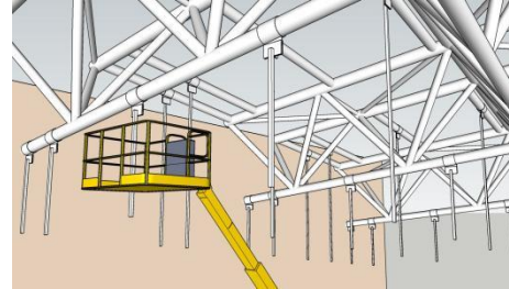
Figure 4 Installation of transfer layer hanger
