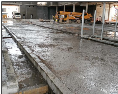
Figure 4 Construction of Slag Concrete Cushion Layer
