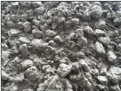
Figure 7 Steel Fiber Concrete
