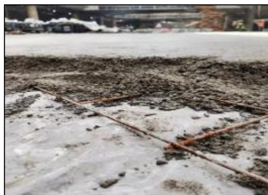
Figure 5 Laying of Sliding Layer
