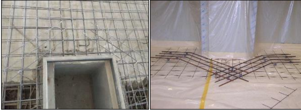
Figure 6 Anti-Crack Reinforcement Setting around Trench and Column
