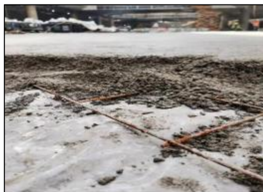
Figure 5 Laying of Sliding Layer
