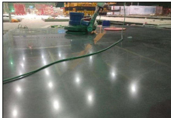
Figure 11 Grinding
