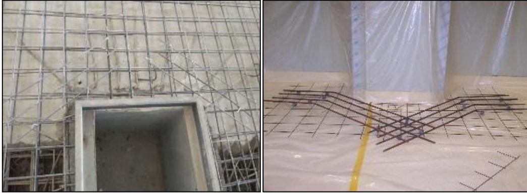
Figure 6 Anti-Crack Reinforcement Setting around Trench and Column
