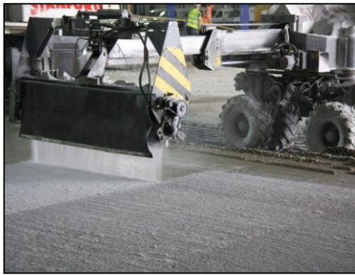
Figure 9 Mechanical Spreading
