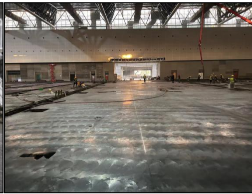
Figure 10 Surface Finishing
