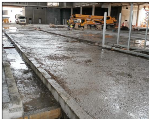
Figure 4 Construction of Slag Concrete Cushion Layer
