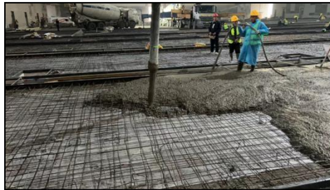
Figure 1 Concrete Pouring
