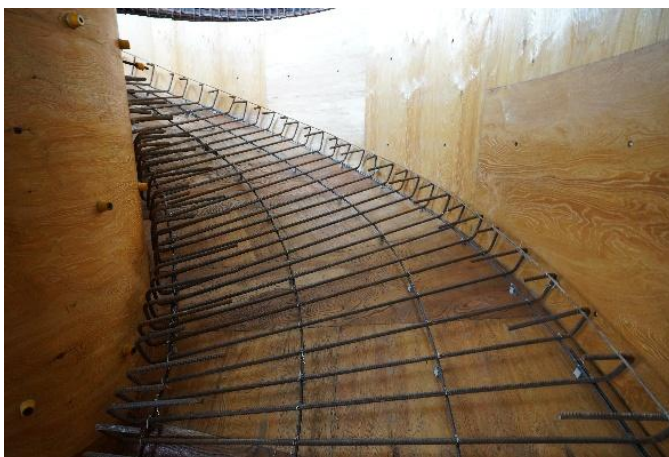
Figure 8 Stair Section Rebar Tying Diagram
