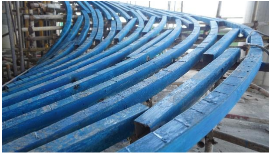
Figure 5 Bottom Formwork Keel Diagram
