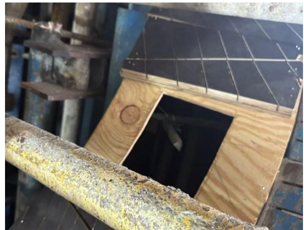
Figure 12 Pouring and Vibrating Opening for the Handrail Surface
