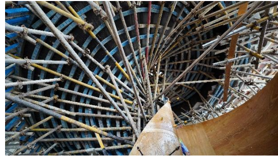
Figure 6 Bottom Formwork Keel Diagram
