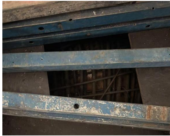
Figure 10 Pouring and Vibrating Opening of the Stair Section Surface
