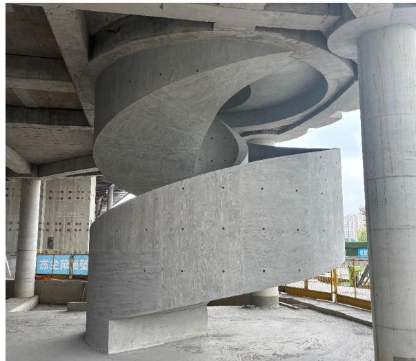
Figure 13 Effect Diagram after Formwork Removal
