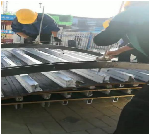
Figure 11 Side Formwork Installation
