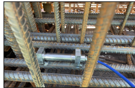
Figure 11 Installation of Beam Stress and Strain Sensors
