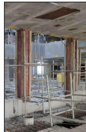
Figure 17 Frame Column Formwork
