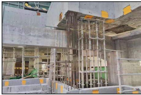
Figure 12 Reserved Longitudinal Reinforcement for the Frame Column
