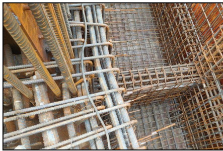
Figure 10 Construction of the Top Floor of the Frame Column
