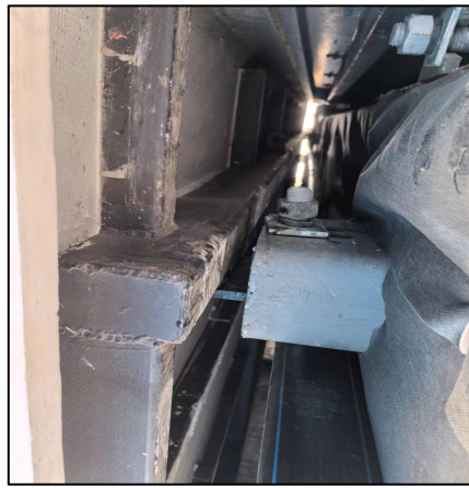
Figure 9 Hanging Plate Leveling and Fixing
