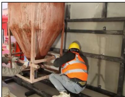
Figure 4 Heavy-duty Hanging Panel Casting
