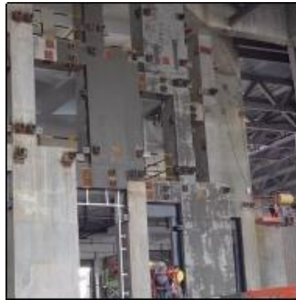
Figure 7 Welding of Bracket Connector
