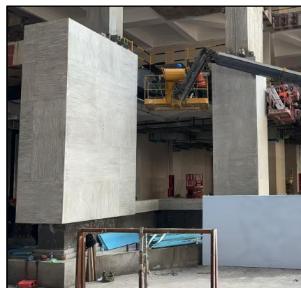
Figure 8 Hanging Plate Hoisting
