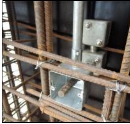
Figure 6 Installation of Embedded Parts
