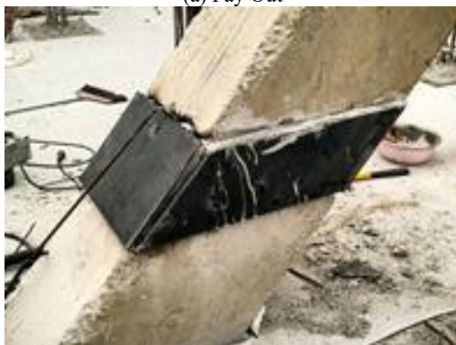
(c) Additional Welding of Angle Iron Batten
