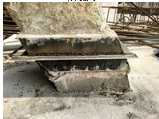
(d) Additional Welding of Waterproof Steel Plate
